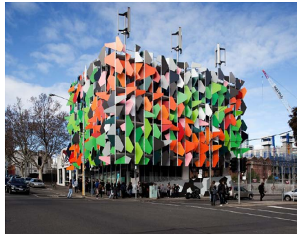
Pixel Building, Melbourne, Australia Designed by Studio 505
